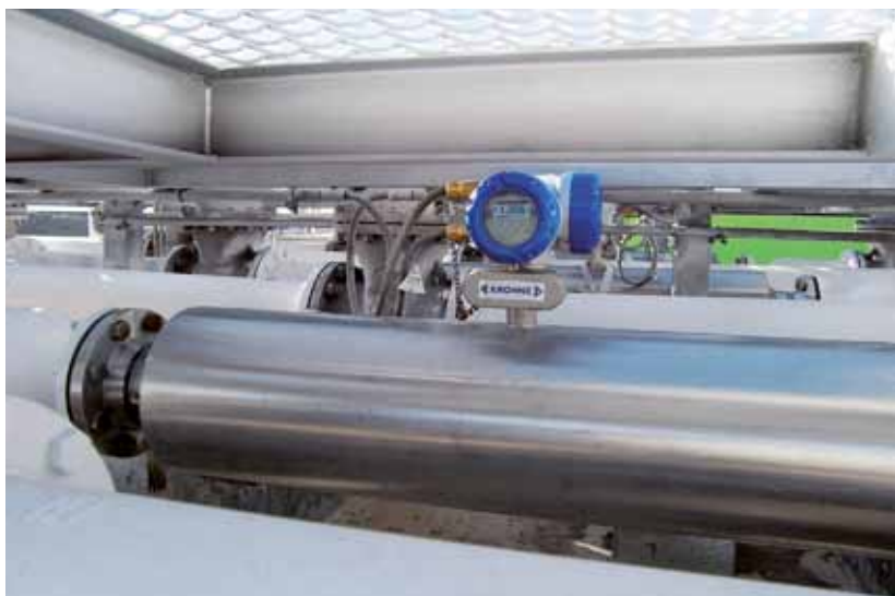
OPTIMASS 2000 – Minimal installation footprint
